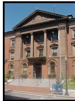
New Bedford City Hall
